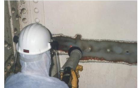
Blast N Vac being used on Steel
